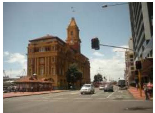
Ferry Building am Hafen
