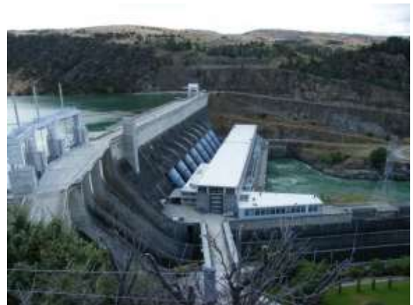
Power Station Roxburgh
