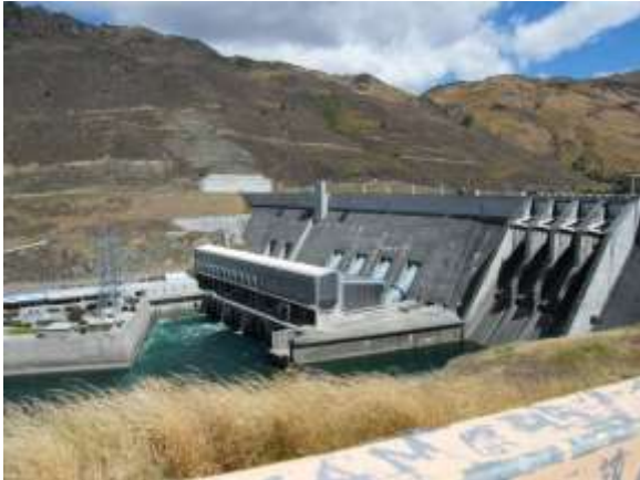
Power Station in Clyde
