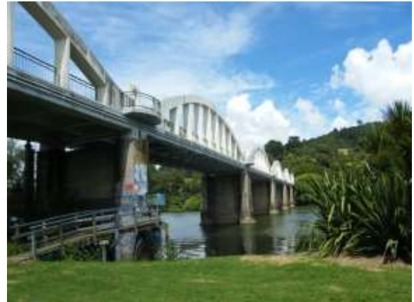
an der Port-Waikato-Tuakau-Bridge-Road
