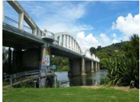
an der Port-Waikato-Tuakau-Bridge-Road
