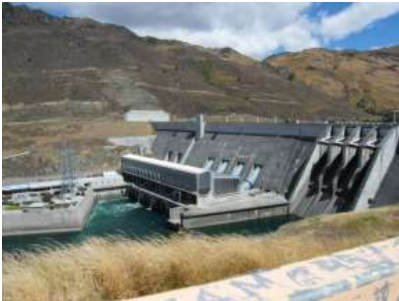
Power Station in Clyde
