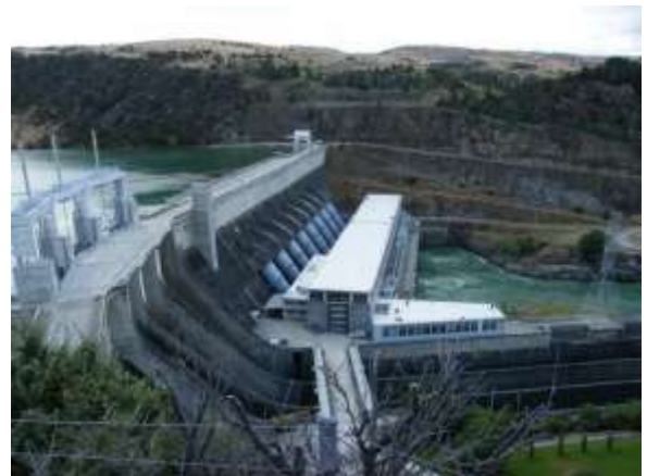
Power Station Roxburgh
