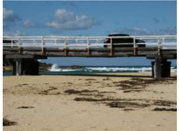
alte One Lane Bridge
